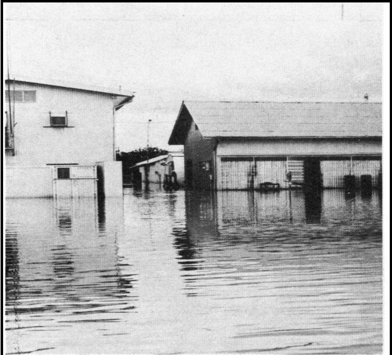
Flood makes a "canal" between Shops/Office building (l.) and Facility Maintenance Shop (r.).
