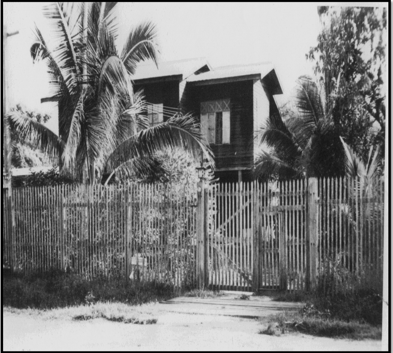
The "Duck House," the raised, wooden, tin roofed structure where Mike Jarina and others lived in Udorn, Thailand.
