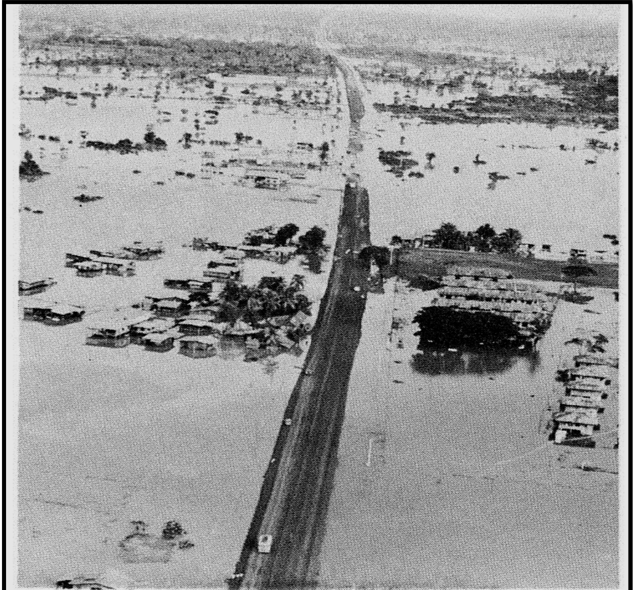
Aerial view of washed out main highway and flooded countryside near Udorn Royal Thai Air Force Base.
