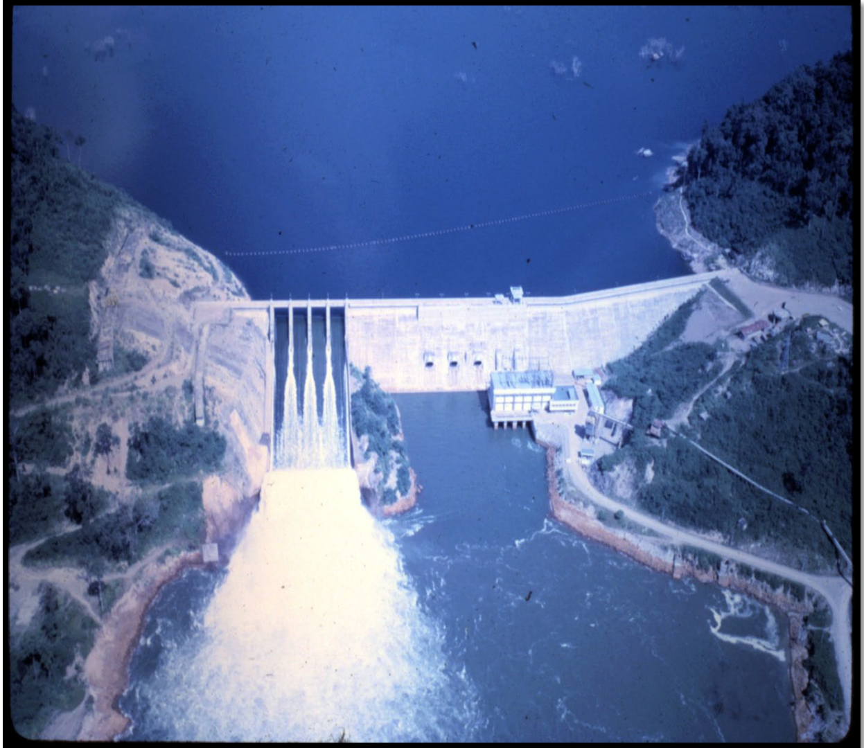
The downstream business portion of the hydroelectric dam on Ritaville's western ridge. The reservoir to the upper portion of the photo contained discharge from the Nam Ngum and its upper reaches. Author Collection.
