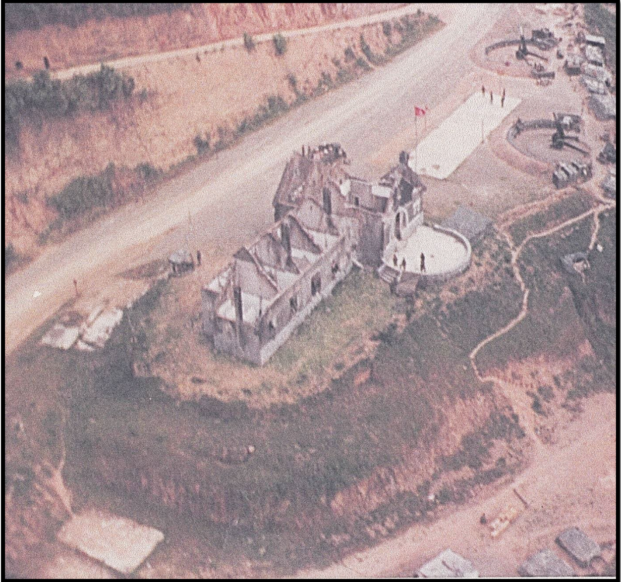
The fortified Sala Phou Khoun Route 7/13 junction (LS-260) during a period of Lao government control following the ceasefire. The shell-shot stone building was originally a French-operated hostel to accommodate travelers between Vientiane and Luang Prabang. Two entrenched artillery pieces are located to the upper right.
