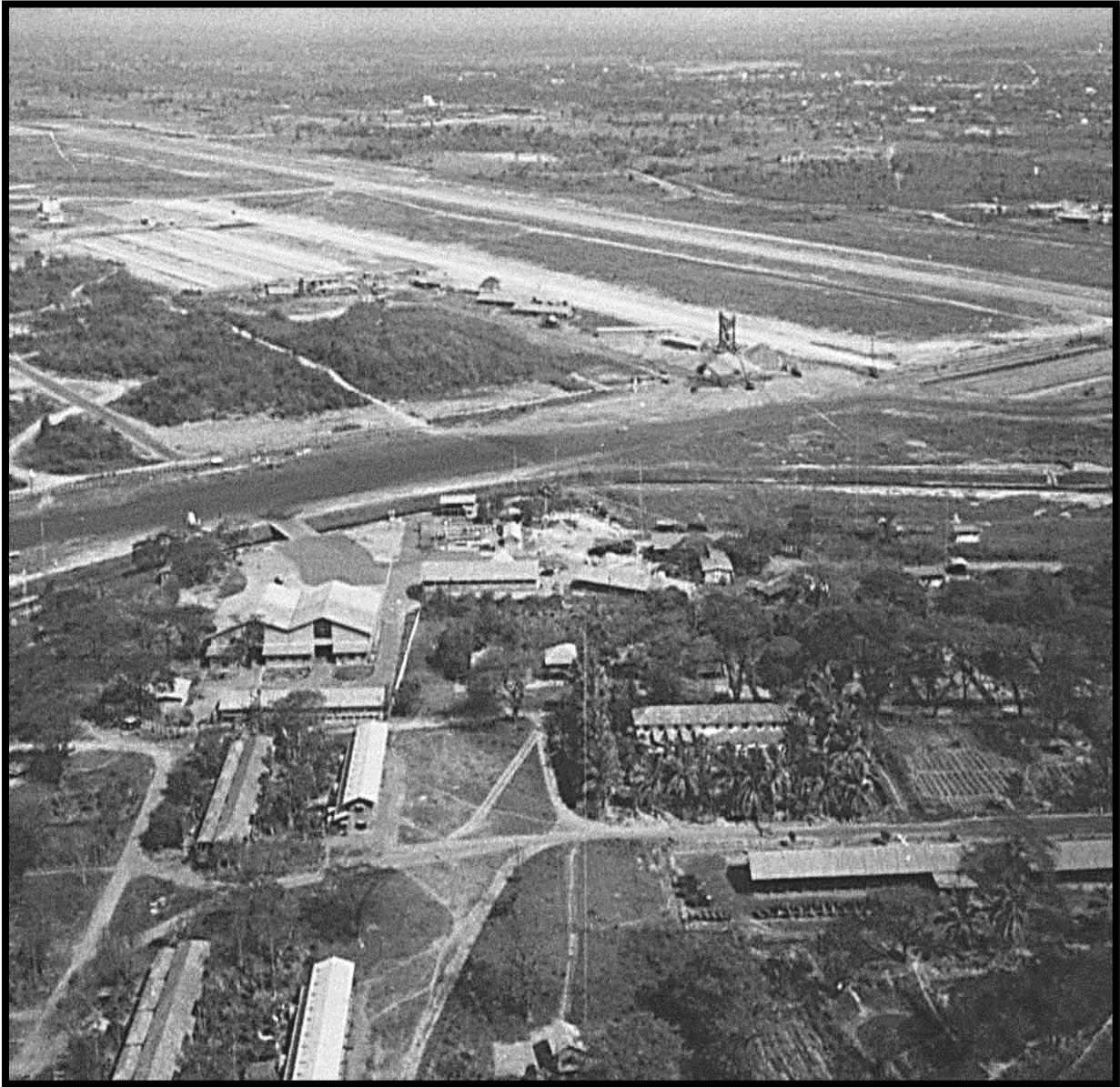
A view to the north from a UH-34D over the Royal Thai Army base of the Air America facility, parking ramp, concrete batching plant, and runway excavation.
