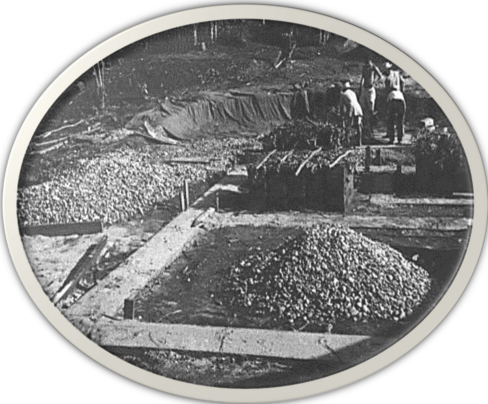
Mud block house footings. Flipse Collection.
