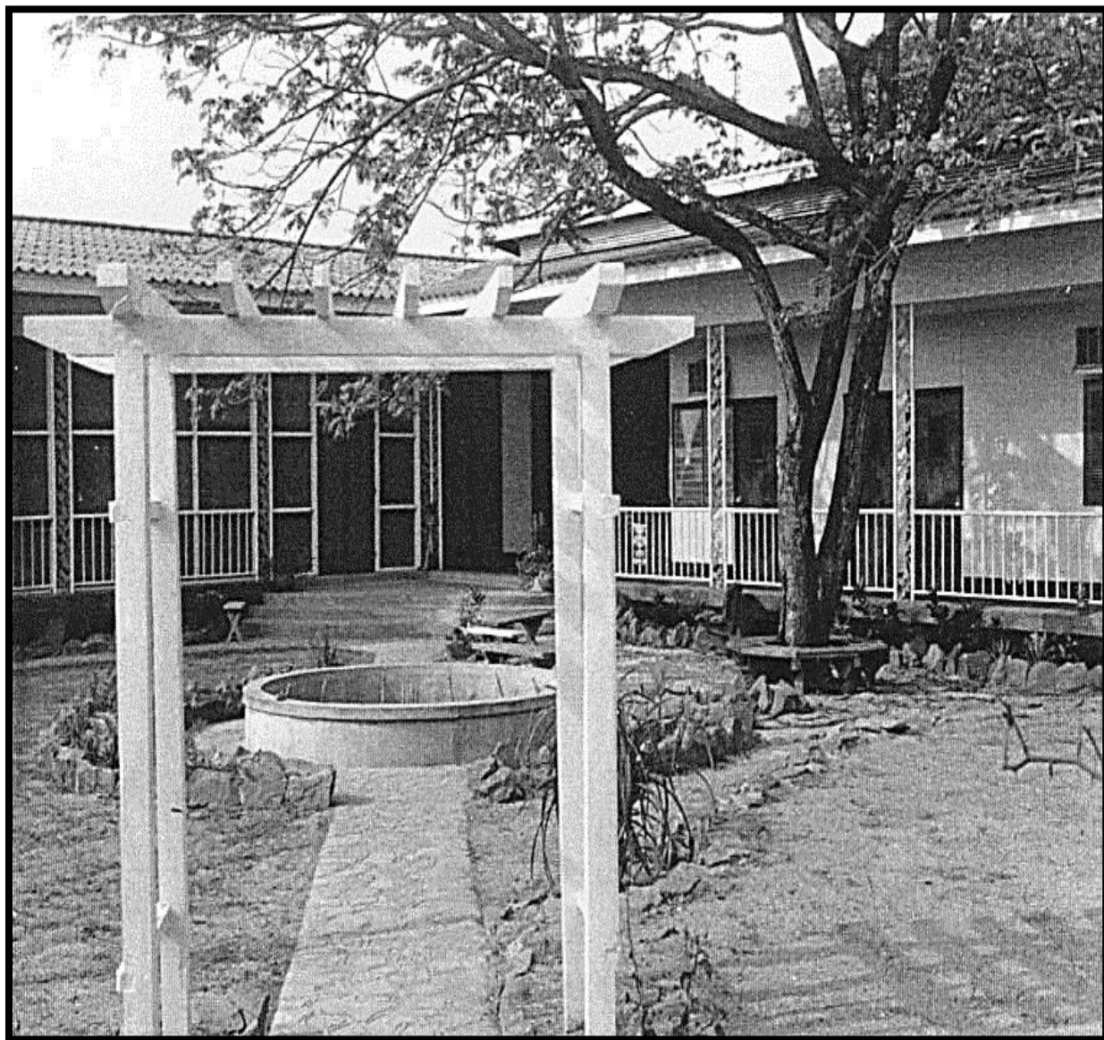
Air America Club displaying the completed fountain, landscaping, and concrete walk between the new Club and the Administration-Operations building.
