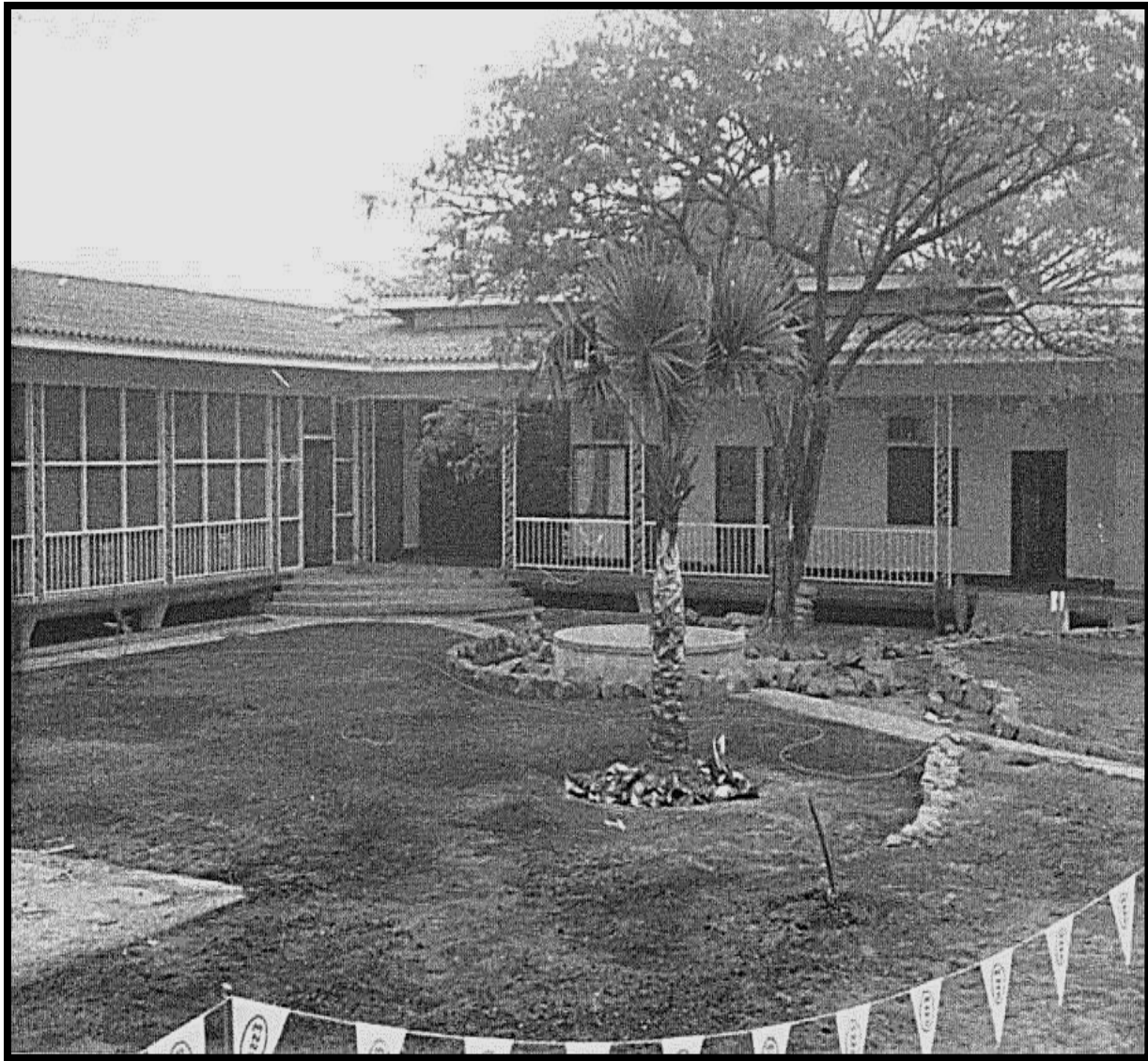
New "L" shaped Air America Club. The screened porch area leads to the dining room. Right portion contains a bathroom, sleeping quarters, and Ben Moore's office.
